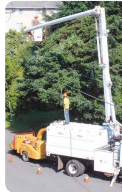
Each year, Newnan Utilities and hired contractors work to trim and remove trees and limbs that pose a threat to electric lines. This work, lasting several months, helps ensure safe and reliable electric service.
